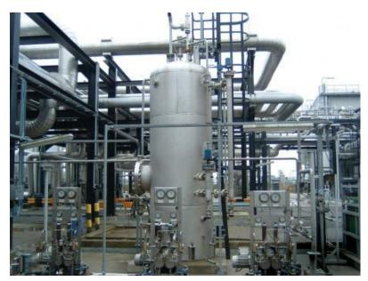
If allowed to be discharged into the atmosphere, the hydrocarbon vapor operating income will be reduced due to the reduction in volume, and it will cause fire hazards and pollution problems. A steam recovery unit (VRU) collects these steams from storage and loading facilities, reliquaries the steam, and returns liquid hydrocarbons to storage. The methods for recovering steam include absorption, condensation, adsorption and simple cooling.
