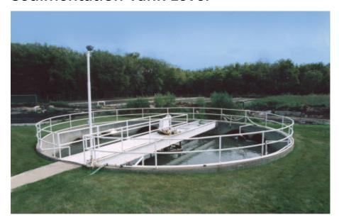
There is only one sedimentation tank in a small sewage treatment facility, and it is necessary to understand the surface level of the sedimentation tank. In larger sewage treatment plants, after the permeated water passes through the diverter box to reach many sedimentation tanks, there may not be enough space in the diverter box to accommodate the level gauge. In this case, the level monitoring of the sedimentation tank will help to obtain proper load balance.
