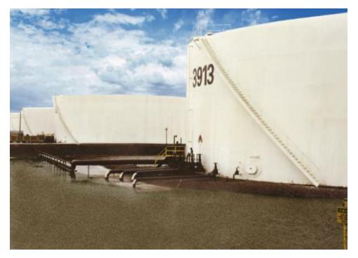
After reaching the refinery terminal, crude oil is pumped into ground storage tanks with storage capacity ranging from thousands to millions of gallons. These tanks are floating-roof or fixed-top tanks manufactured on site according to API standards.
