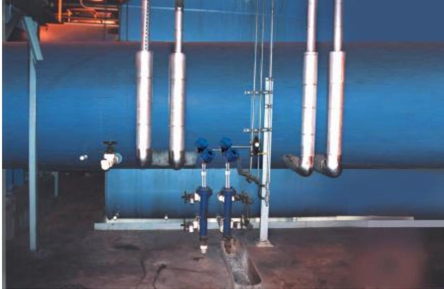
Vapor enters the condenser to cool and condense into water before entering the low-pressure feedwater heater. The condenser hot well serves as a reservoir for turbine circulation. When the level in the hot well reaches its lowest point, a valve opens to provide recharge water for circulation. When the hot well level reaches the high end of the range, the drain valve is opened to drain the condensate from the hot well to the condensate tank.
