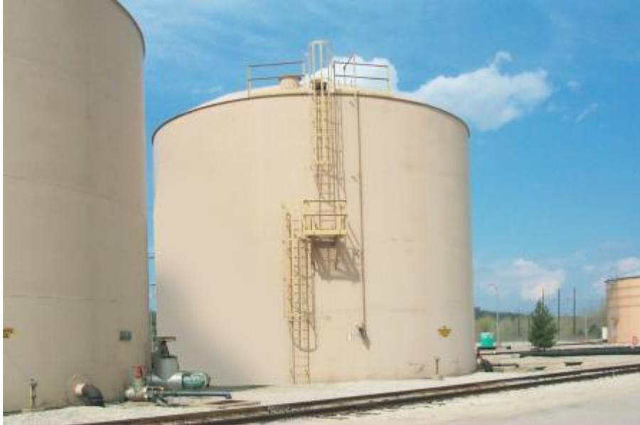
When the condenser hot well level reaches a high point, the drain valve opens, draining excess condensate from the hot well to the condensate storage tank. As condensate is lost in the turbine cycle, the hot well level drops, at which point the water supply valve in the storage tank is opened to provide supplemental water for the Condenser hot wells.
